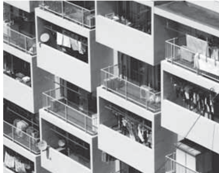
Housing densities, which vary by country, culture and region, as well as economies, can have a range of impacts on both health and environment. Pictured here is an apartment building in Nagoya, Japan. (Photo: Andrew Martin)
