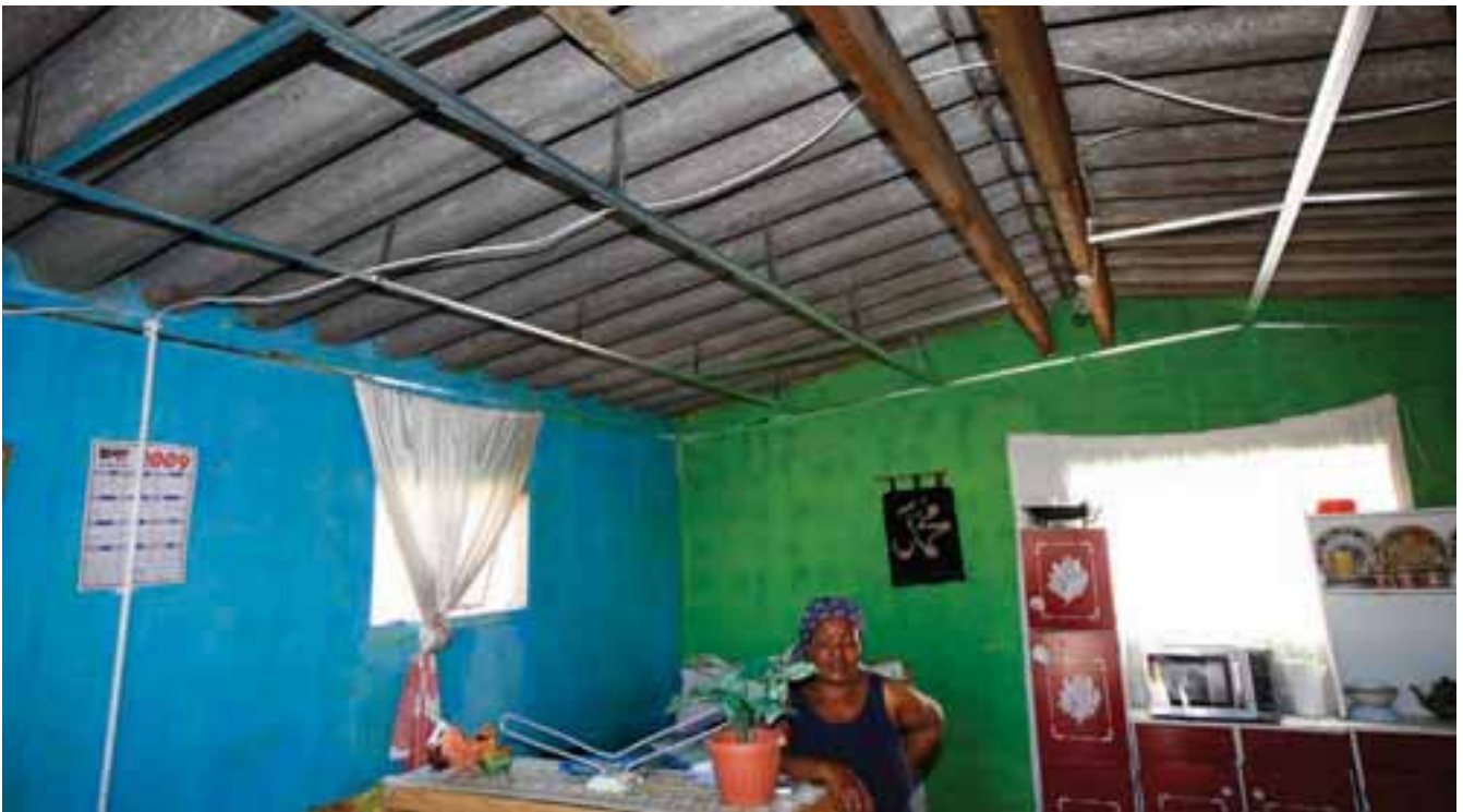
A typical Kuyasa interior, prior to retrofit. The exposed tin roof radiates heat in the summer and absorbs cold and moisture in the winter. Ceiling insulation being added as part of the improvements should help reduce damp and temperature extremes, and save energy. (Photo: Nic Bothma, Kuyasa/CDM Project)
