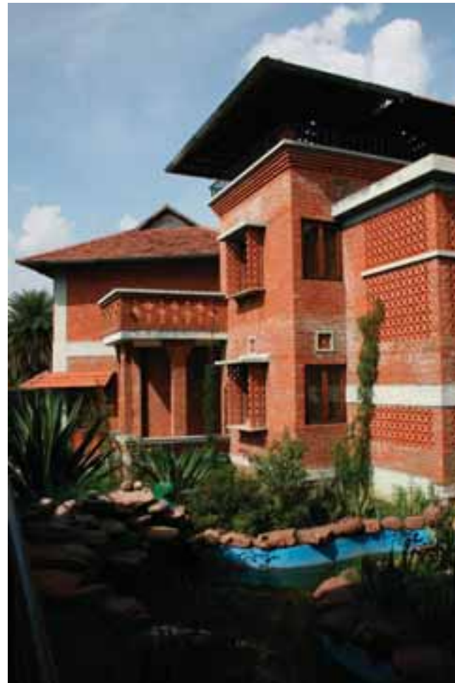
Lattice work and air flow under the roof eaves illustrates modern use of traditional natural ventilation features. (Photo: Maude Dorr)
