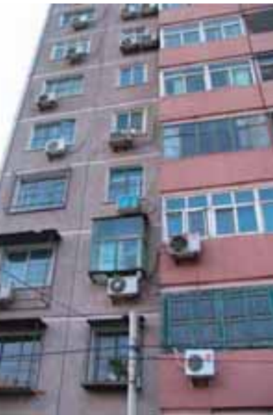
Air conditioners in a building in Beijing, China. (Photo: Matthias Braubach)
