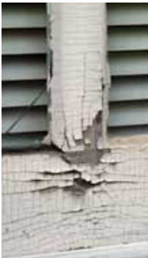
Old paint can contain lead, which is toxic to humans and especially dangerous to children. (Photo: istockphoto)
