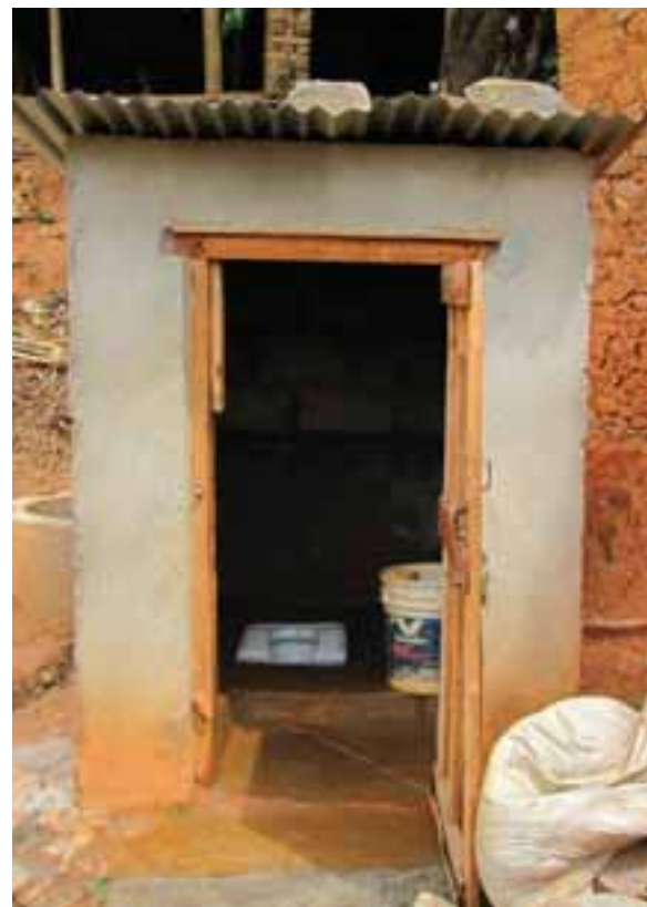
Biogas latrine built as part of a clean fuel project undertaken by “the World in Justice” NGO in a village of rural Nepal. The health benefit is three-fold: improved access to sanitation through the latrine hookup, reduced indoor air pollution from the use of biogas for cooking; and reduced climate change through use of a renewable fuel source. (Photo: Heather Adair-Rohani)
